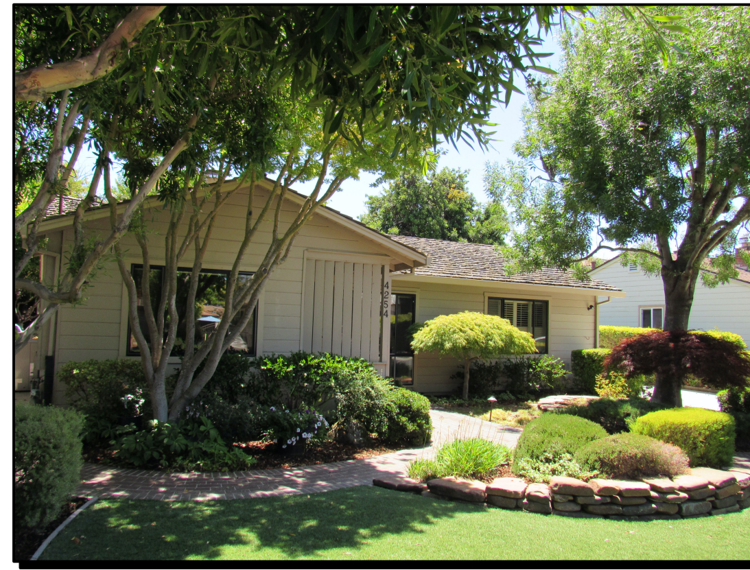
EXISTING SITE PHOTO
